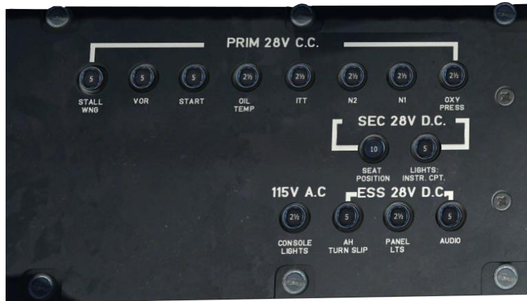
Figure 9-9 Rear Circuit Breaker Panel
