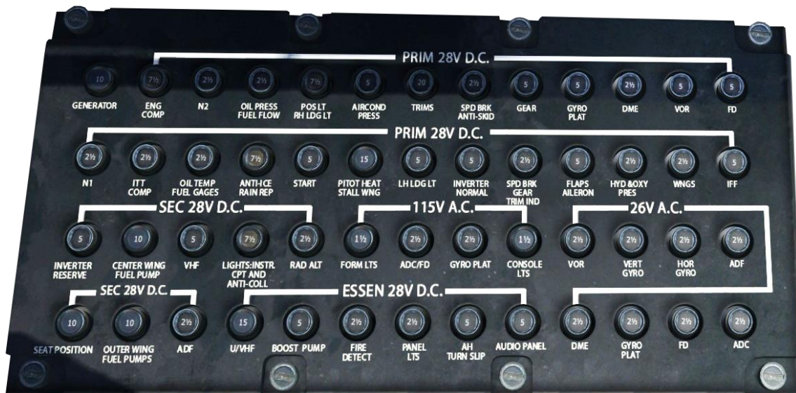
Figure 9-8 Front Circuit Breaker Panel
